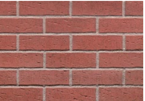
Brick tower (HF03)
